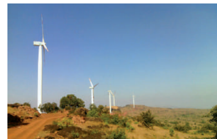
Wind Power Plant
