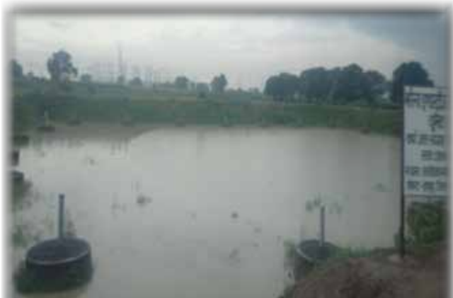
The Achheja Gaon pond constructed and Maintained by Merino for ground-water recharge
