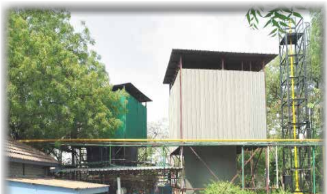
Biogas plant in MIL- Hapur
