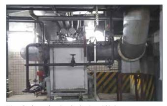
Water Pre-heater housing the ducting within its core
