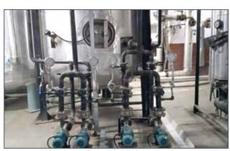
Circulation pumps with standby for hot water movement to swimming pool and rooms heat exchanger
